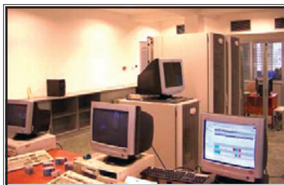
New Server Room
