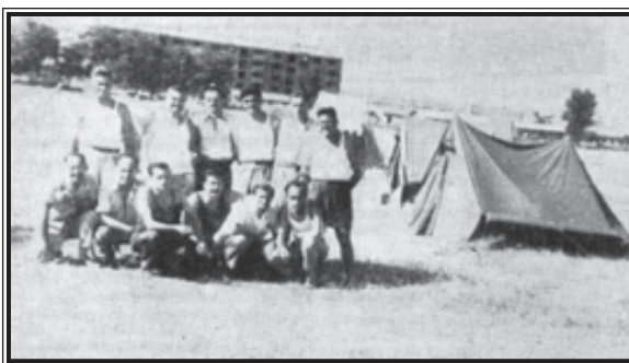
Customs House Skopje under tents – immediately after the earthquake on 26 th July 1963
