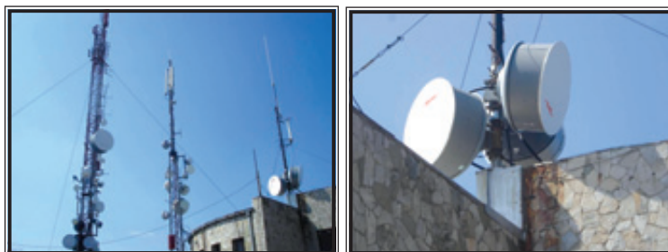
Radio equipment Antennas, part of the SDH network
